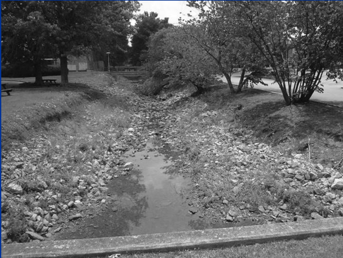
A channelized stream in poor condition
