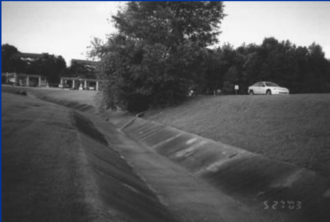
A concrete trapezoidal channel
